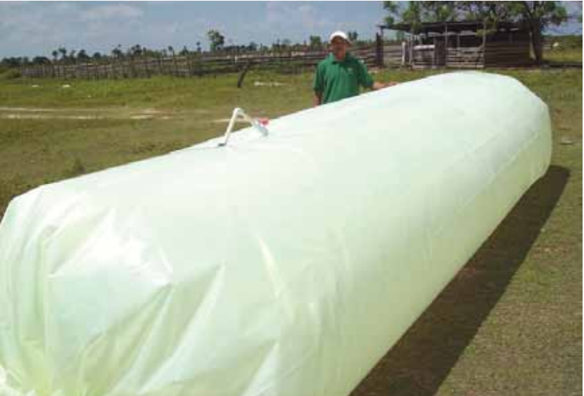
Figure 7: A biodigester being installed (Lethem)
