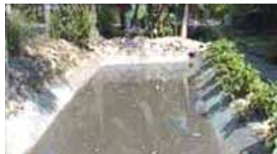
The pond ready and full of water (next day)
