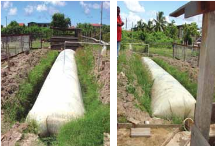
Figure 8 & 9: A biodigester being installed (Berbice)
