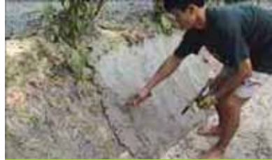
Putting the mixture on the walls of the pond
