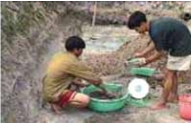
Mixing the soil and cement
